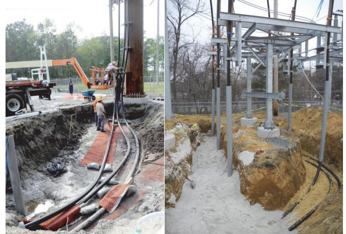
Figure 7: Direct buried section near a compact transition pole with one cable per phase (left) and conventional risers with two cable per phase (right)
