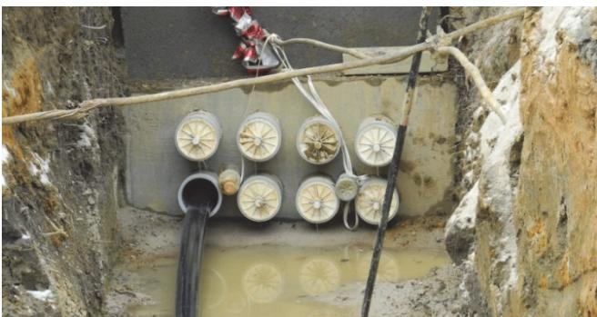
Figure 5: 2x4 duct bank, with 6-in conduits and 9-5/8in center-line separation
