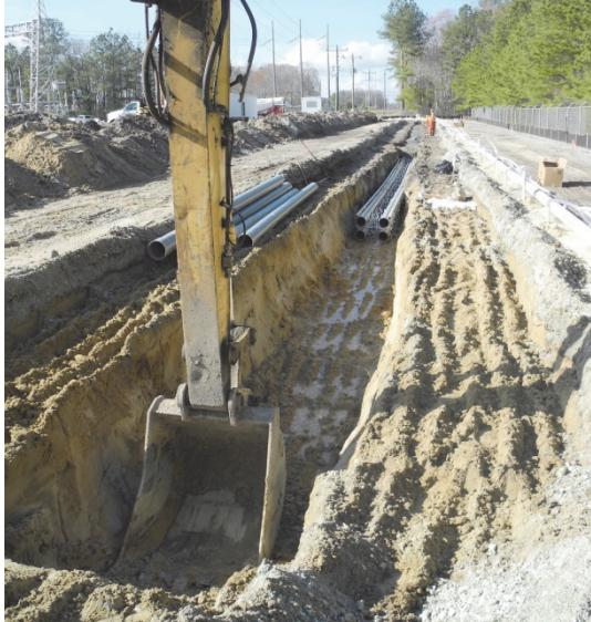
Figure 4: Open cut excavation
