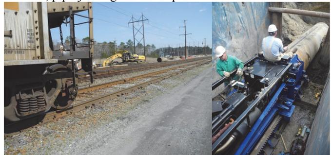
Figure 8: Pipe-jacking operation under rail sidings
