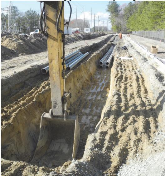
Figure 4: Open cut excavation
