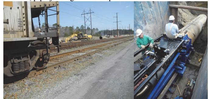
Figure 8: Pipe-jacking operation under rail sidings
