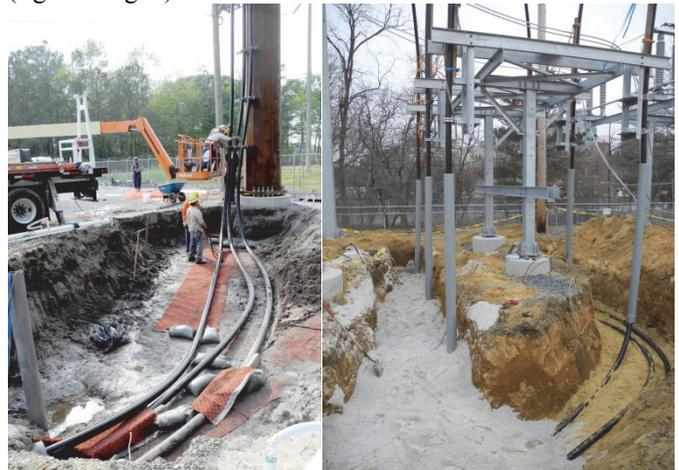
Figure 7: Direct buried section near a compact transition pole with one cable per phase (left) and conventional risers with two cable per phase (right)
