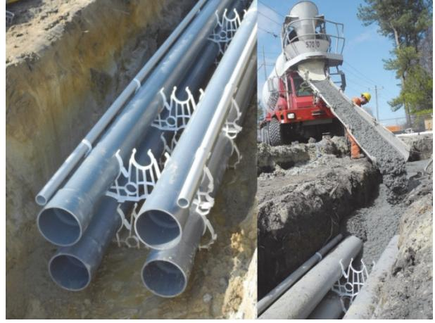
Figure 6: 2x2 duct bank (left) and concrete backfill installation (right)
